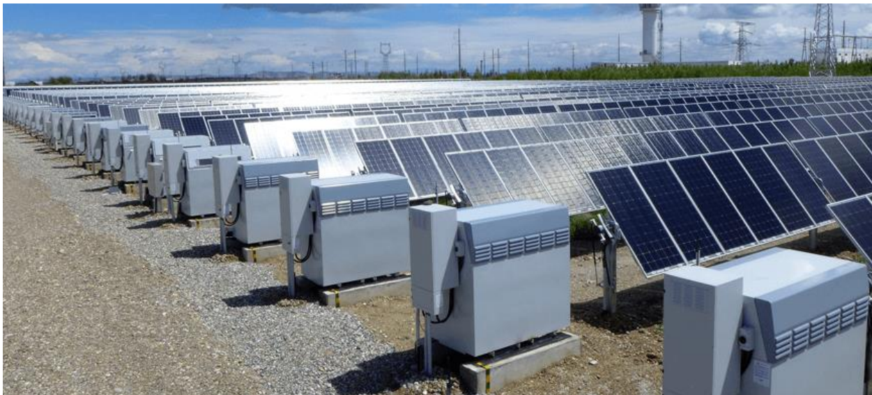
A NEXTracker's NX Flow™ integrated solar-plus-storage system. Image: Courtesy of NEXTracker
