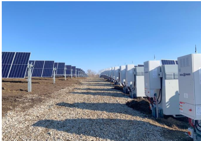
A NEXTracker's NX Flow integrated solar-plus-storage system with DC-coupled NEM energy storage. Image: Courtesy of Ideal Energy
